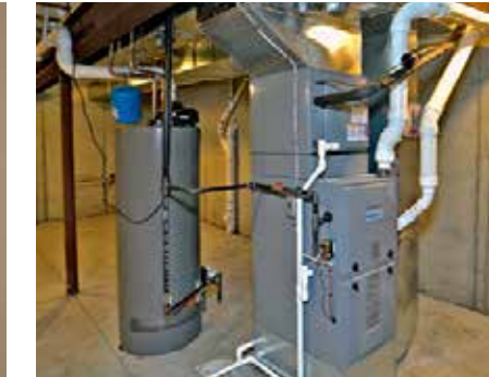
95% High efficiency gas furnace with add on humidifier (10yr warranty - parts & labor)
