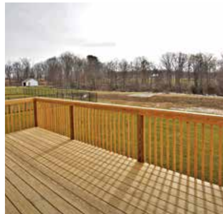
Uncovered Wood Deck
