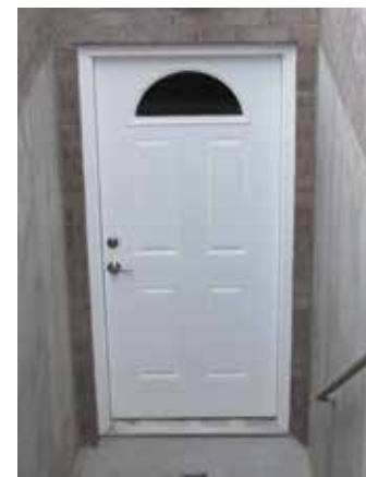
Single Basement Exit Door
