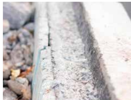
Foundation walls back filled with crushed stone
