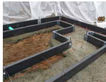
Form-a-drain with stone back fill
