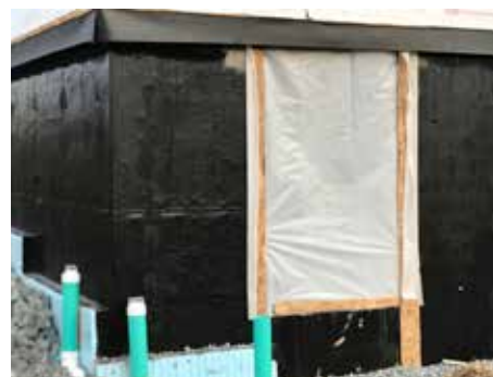
Foundation waterproofing system with expandable tar and 1" styrofoam
