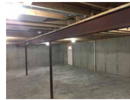
2" x 10" floor joists on 16" center and Steel I-beams
