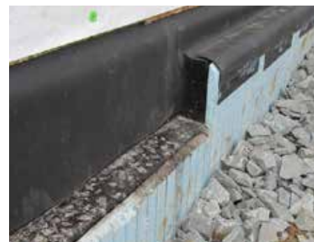
16" rubber water flashing behind brick
