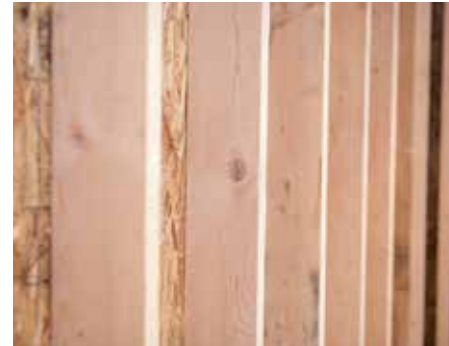
2" x 6" exterior studs on 16" center
