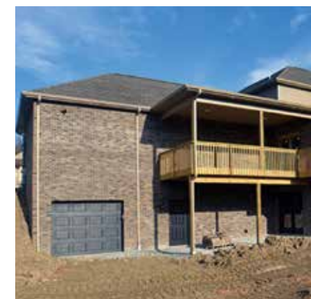
Excavate Under Garage
