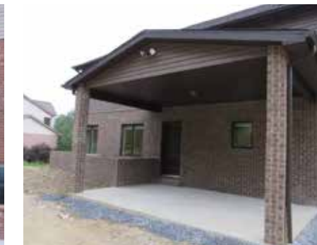
Covered rear deck *or* concrete patio per design & Lot Grade. Classic Series Only.
