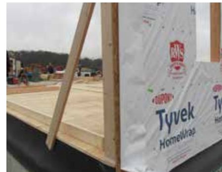
7/16" OSB board exterior walls
