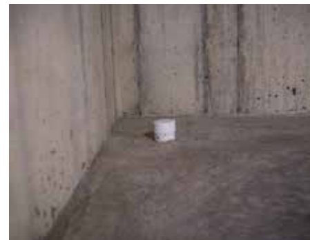
Interior and exterior french drains
