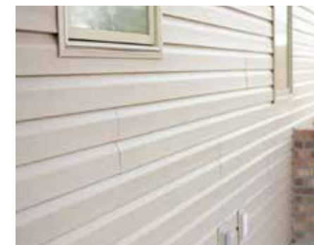
Vinyl siding on non-brick areas
