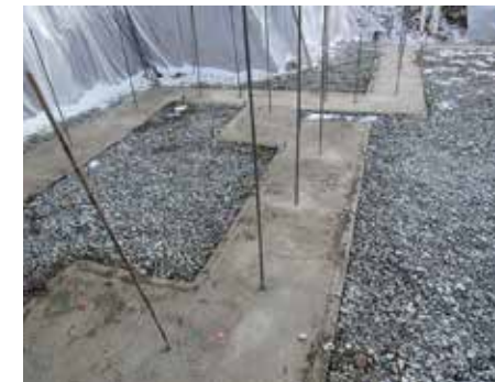
20" poured 4,000 concrete footer with rebar (RWS does not use gravel footers)
