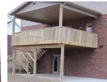
Covered rear deck *or* concrete patio per design & Lot Grade. Classic Series Only.
