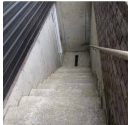
Exterior Basement Steps
