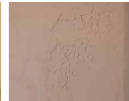
Hard-coat plaster with textured finish
