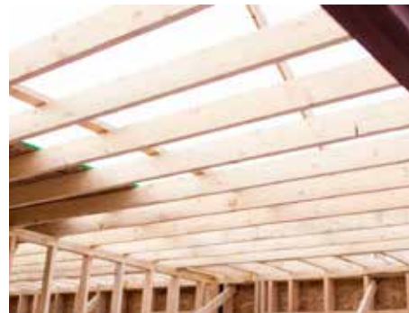
2" x 6" rafters on 16" center or trusses
