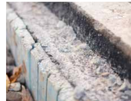
Foundation walls 10" poured 4,000 pound concrete with 1/2" rebar
